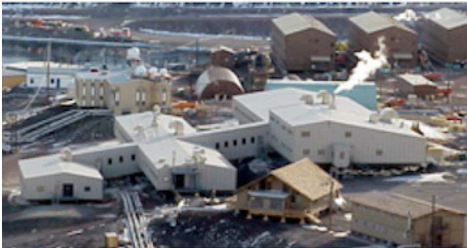
Albert P. Crary Science and Engineering Center, 1991
